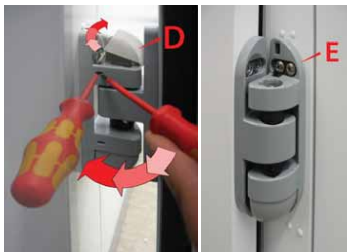
Pic. serie 13. Assembly of the hinges
